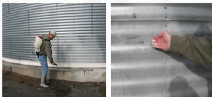
Painting exterior of grain storage facility takes only minutes. A back pack sprayer is used for this small silo. For large jobs an agricultural sprayer would be more effective.
