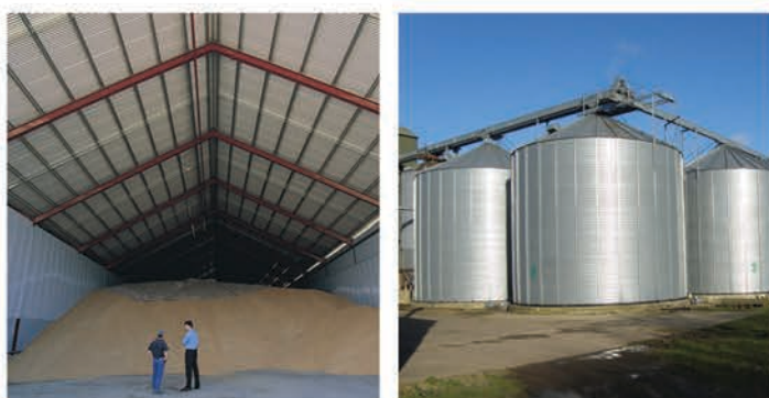
Custom Integrated Pest Management Solutions for all types of Storage Facilities
