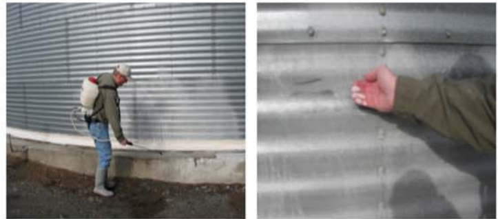
Painting exterior of grain storage facility takes only minutes. A back pack sprayer is used for this small silo. For large jobs an agricultural sprayer would be more effective.
